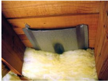
Place rafter vent baffles in between the rafters (DOE photo)
